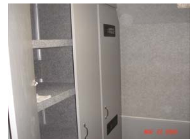
Storage and Power Panels
